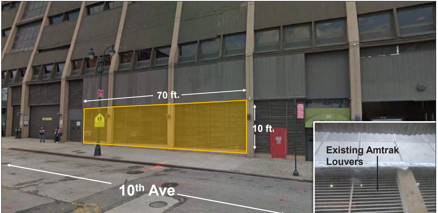
Existing louvers to be used by new Tenth Avenue fan plant 2
